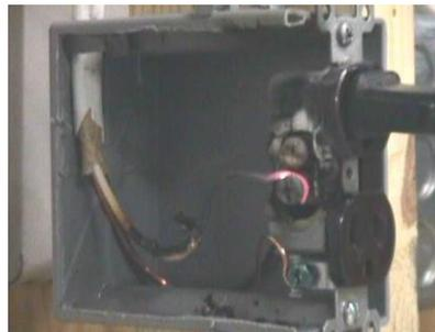
Fig. 6 Glowing contact on duplex receptacle neutral terminal
